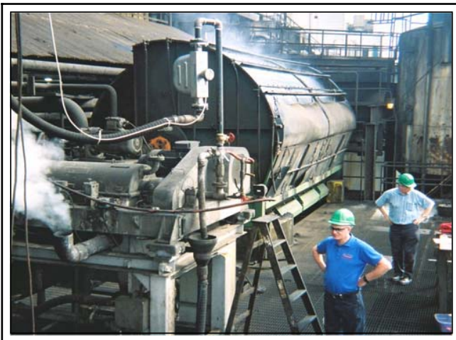
Small scale decanter site trial prior to full scale installation.
